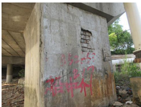
2-1#墩严重胀裂锈蚀
