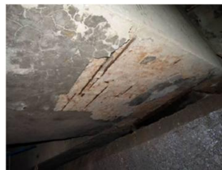
2-2#系梁底露筋锈蚀
