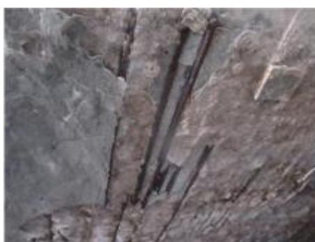
5-2#系梁底面锈胀露筋
