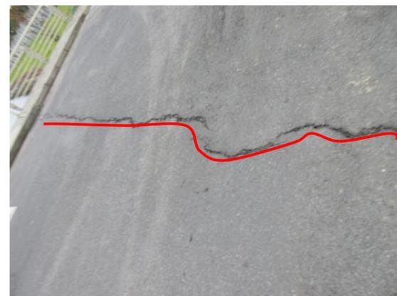
(b) 桥面铺装横向裂缝
