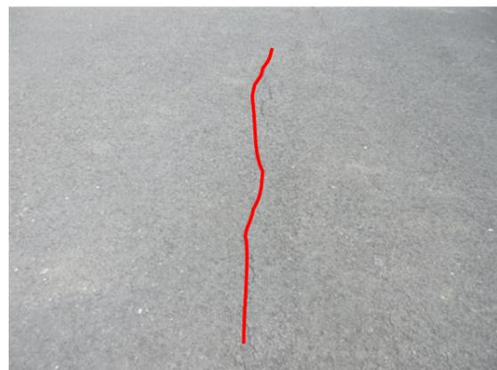
(a) 桥面铺装纵向裂缝
