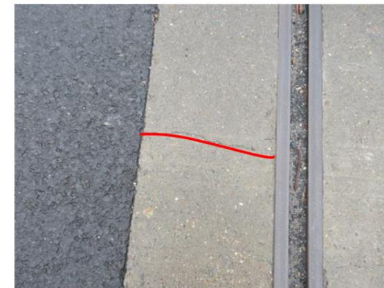
(h) 锚固区纵向裂缝
