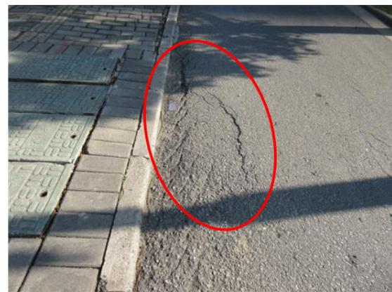
(c) 桥面铺装网状裂缝
