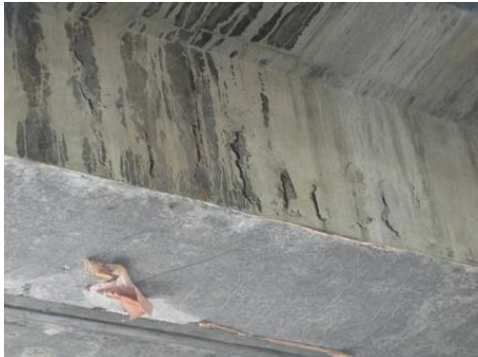
(c) 6-15#梁右腹板锈胀，露筋
