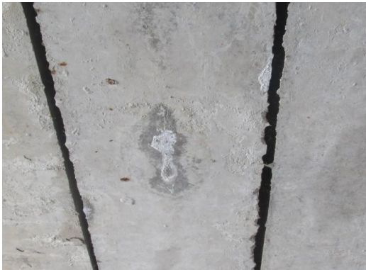
(c) 1-21#梁底板纵向裂缝，析白
