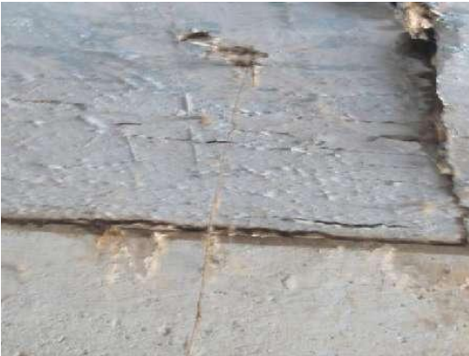
(a) 1-2#梁底板锈胀，露筋锈蚀
