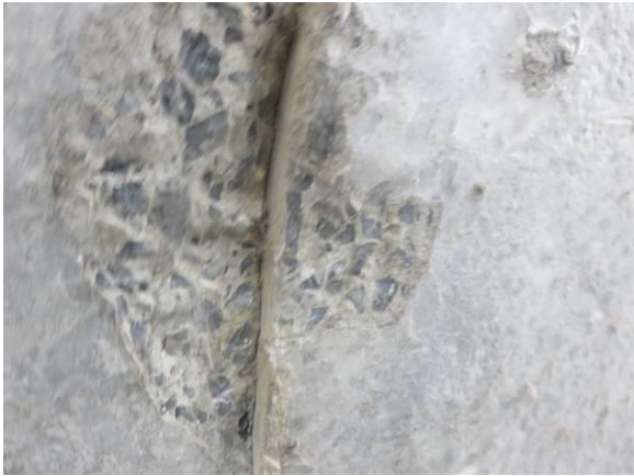
2-12#梁底板破损
