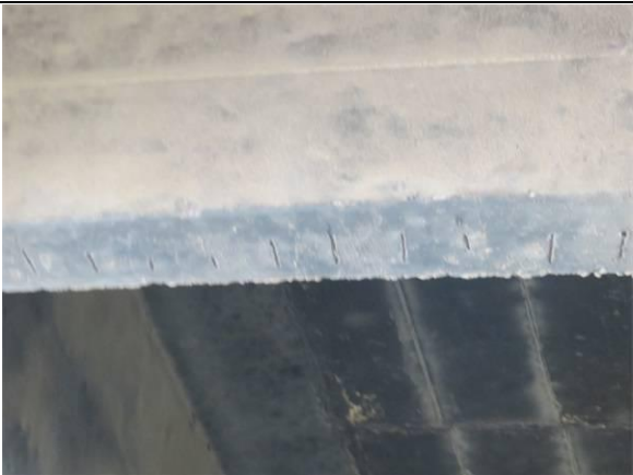
1-6-2 露筋锈蚀
