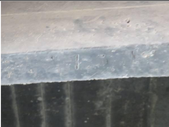
1-4-2 露筋锈蚀
