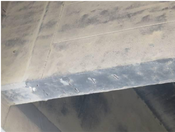
1-7-2 露筋锈蚀
