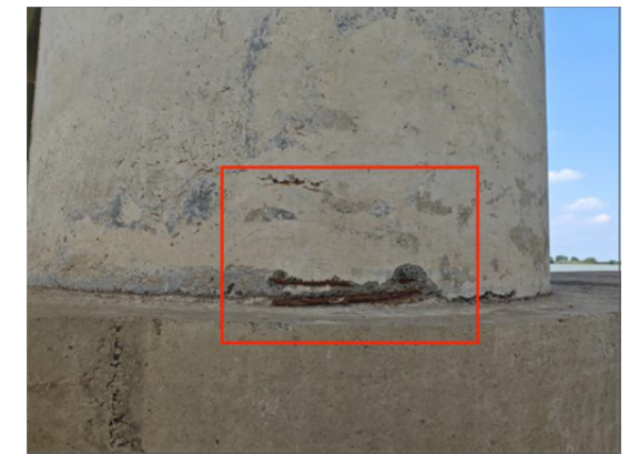
63-2#墩锈胀露筋
