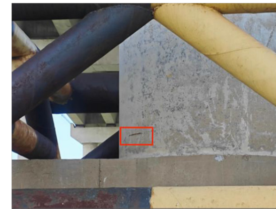
45-1#墩锈胀露筋
