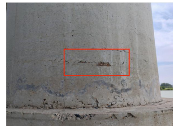
69-2#墩锈胀露筋
