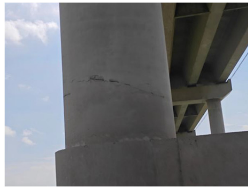
42-1#墩锈胀露筋
