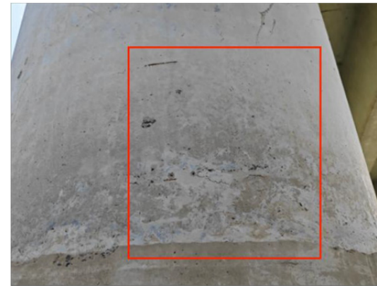
59-1#墩锈胀露筋
