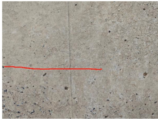
63-2#系梁裂缝
